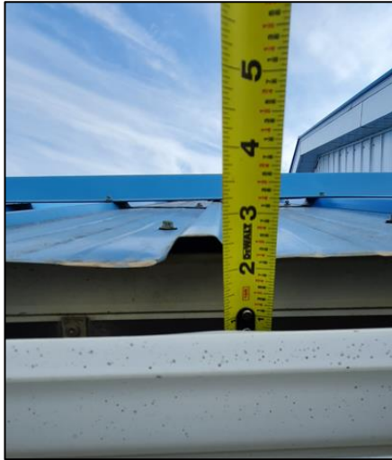
Figure 7 – Corrugated Metal Trapezoid Dimensions
